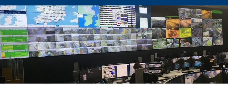
Operational 24/7, the Motorway Traffic Control Centre receives multiple live data feeds from Dublin's road and tunnel network. A vast 15 metre long NEC video wall provides operators with instant access to information as they maintain safe and efficient traffic management.
